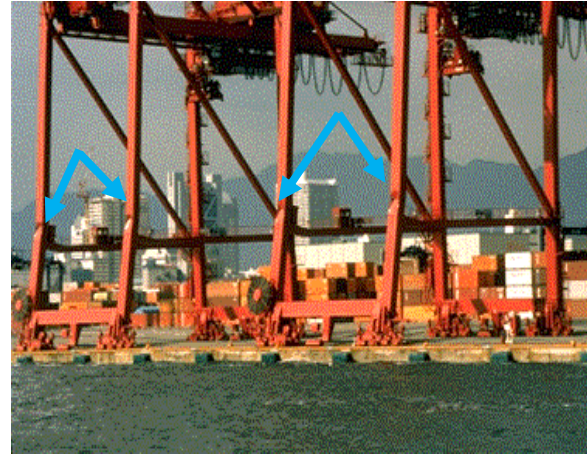
Figure 3.11 Plastically Yielded Crane Legs due to Inadequate foundations [18]
