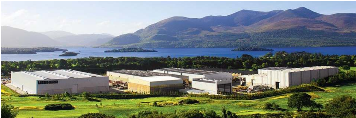
Figure 2.1 Liebherr Plant, Killarney, Co Kerry, Ireland [1]
