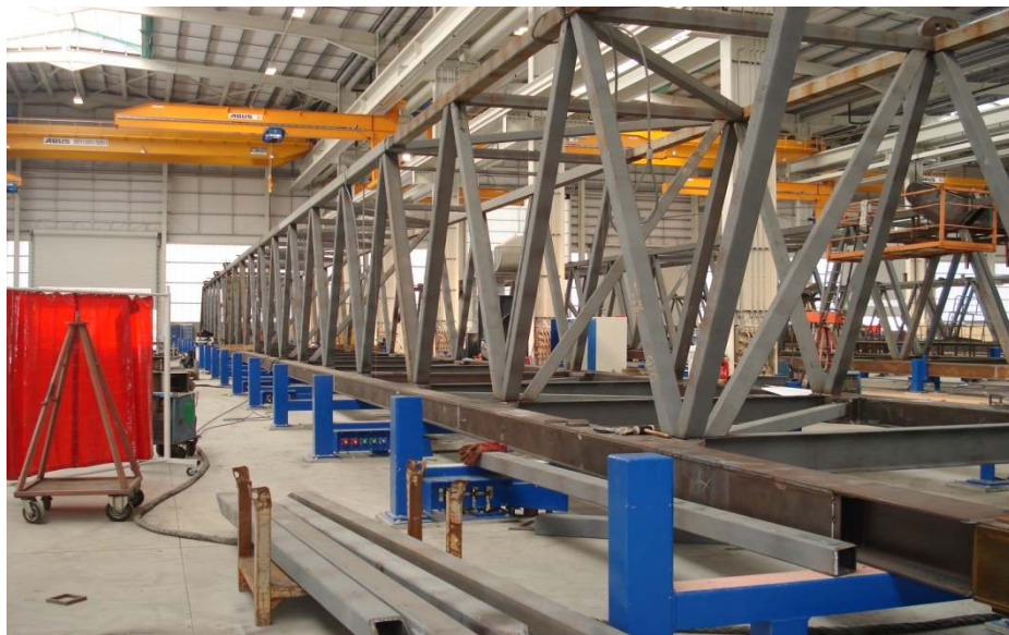
Figure C8 Crane Structural Geometry- Photos by B.Hand
