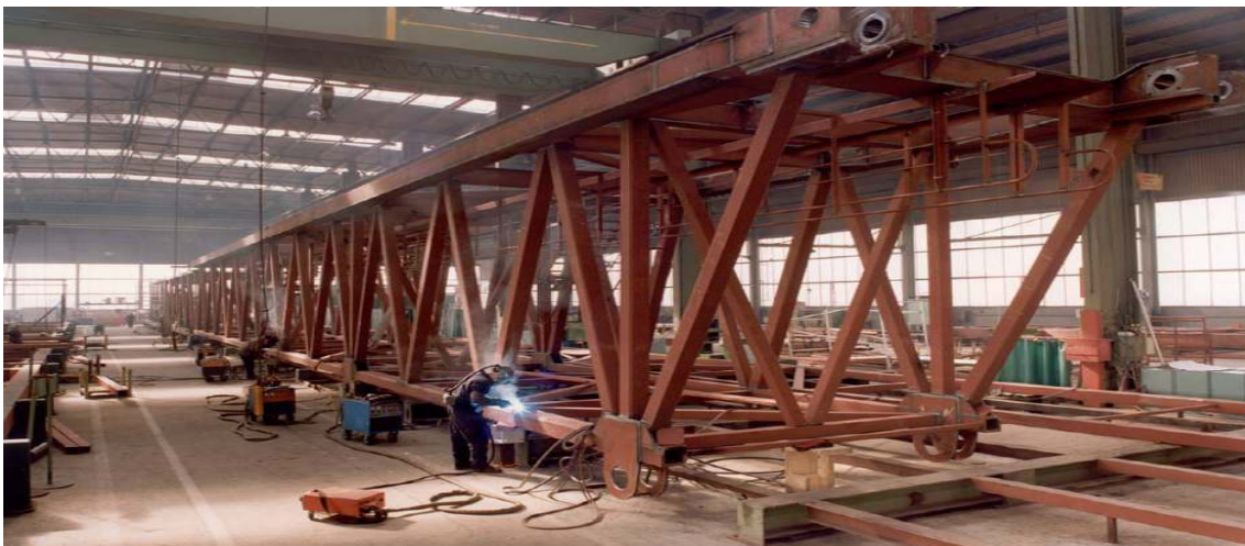
Figure 4.4 Crane Derrick Boom Structure – Photo by B.Hand 2013
